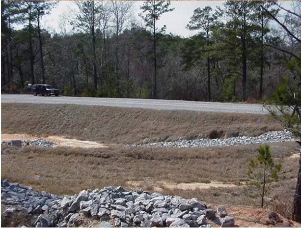
F3. Road was stabilized and banked. A sediment catchment basin was created and hillslopes were stabilized with vegetation and rip-rock. Project was completed in June 2005.
