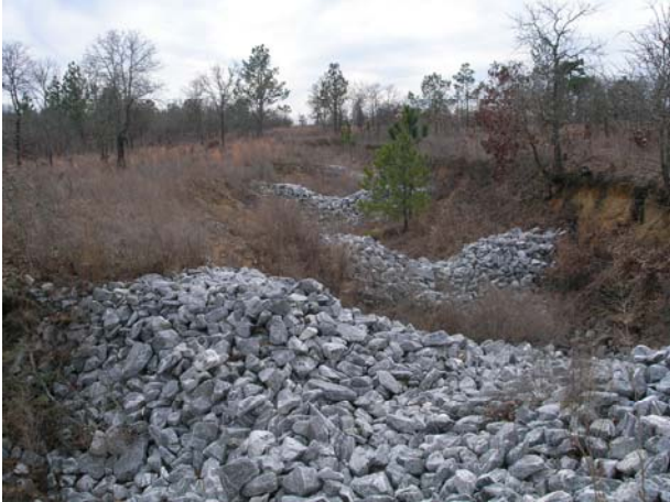
K11E. Erosion gullies were stabilized with rip-rock and grasses and trees were planted in surrounding areas. Project was completed in July 2004.
