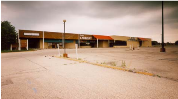
Figure 1: Former dry cleaning facility (pre-redevelopment).
