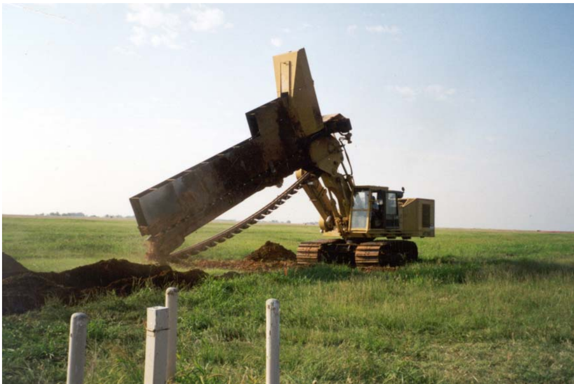
Figure 5.7 Continuous Trenching for Biowall Installation, Altus AFB, Oklahoma
